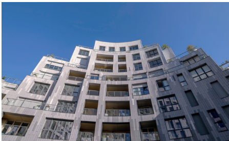
The exterior façades curve and the interior façades are cut to provide as many terraces as possible.
