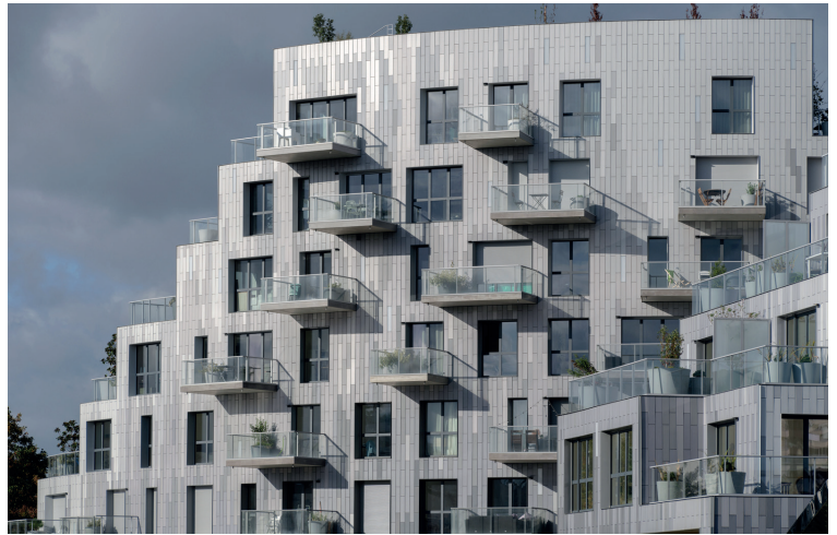
KeraTwin by Agrob Buchtal envelops the project in a colour gradient from grey to white, with a texture from matt to glossy, creating the impression of rock.
