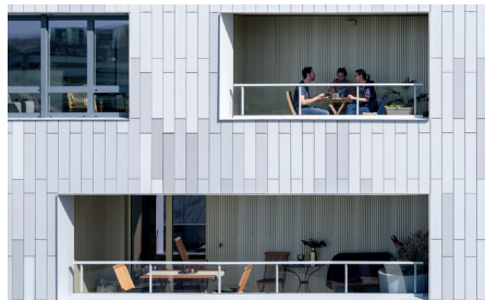
The envelope offers different types of outdoor spaces for the flats: Winter gardens, loggias, balconies and generous terraces also contribute functionally to shading, as privacy screens, noise protection and windbreaks.
